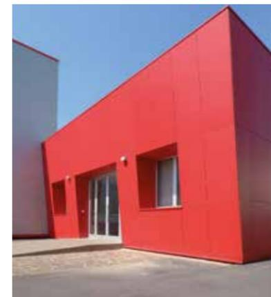
Photo of new facade with ArkWall System panels
