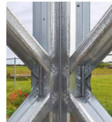
Photo with Wind bracing and vertical profile (detail 3)
